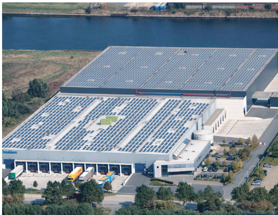
Top: A 428.4 kWp solar installation by Enfinity atop the sloped rooftop of Van Cauwenberge, a family-run lumber business in Zottegem, Belgium. Courtesy of Enfinity Canada Ltd.
